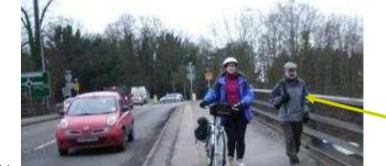
Motorway Bridge Parapet needs to be raised by 300mm.
