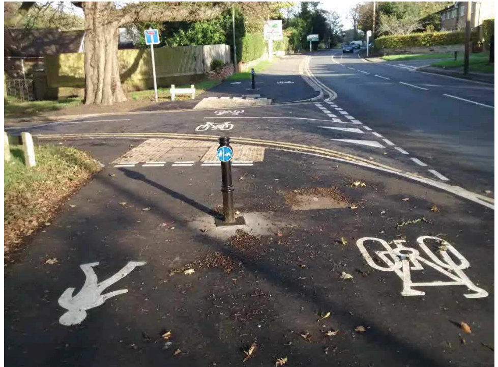
Bollards in the middle of the path (entrance to Homelands)
